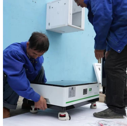
Utility-scale battery energy storage system (BESS)
